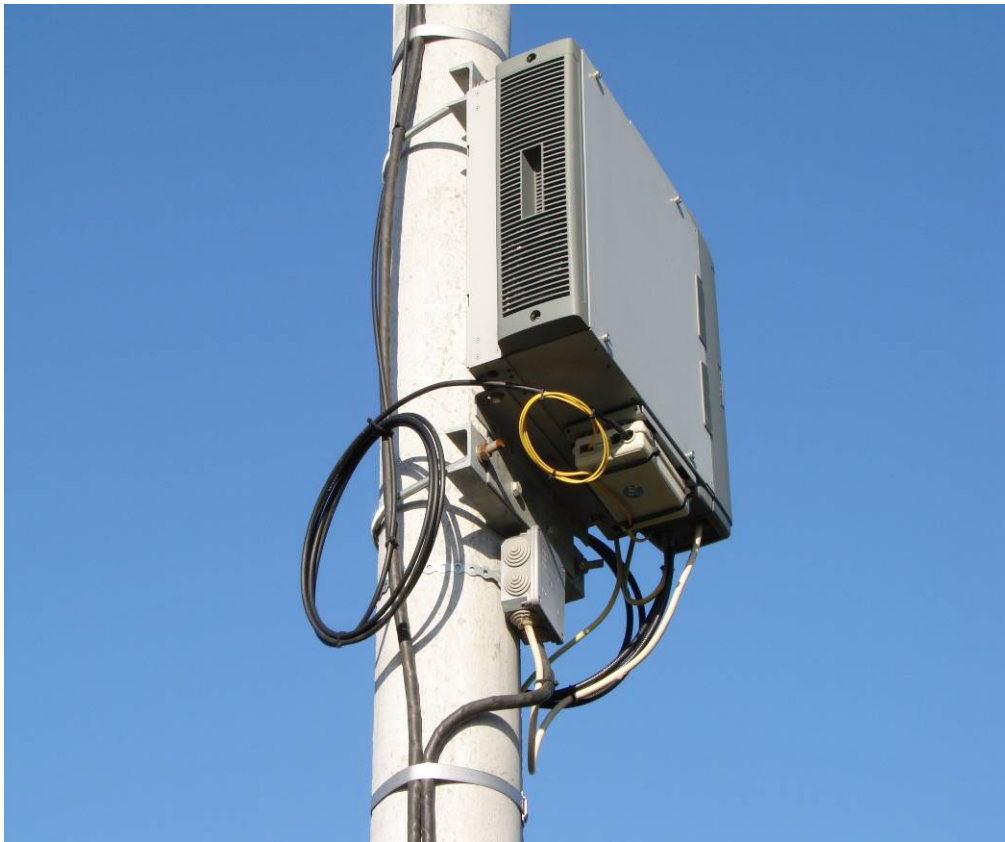
Figura 2.20. Echipament Nokia Flexi BTS
